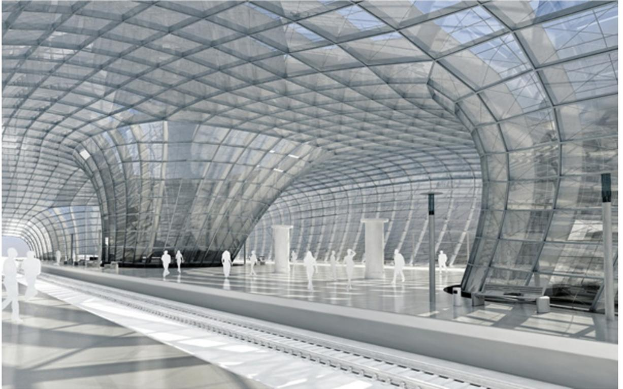
**Figure 7** This mesh which possesses a face-face offset at constant distance has been created by an iterative design process which employs subdivision and optimization using both (2) and (3) in an alternating way (image courtesy B. Schneider).
